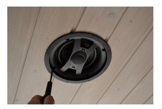
**Fig 15.** The speaker unit is screwed into the ceiling so that the 4 "dogear" brackets in the device are fixed to the cabinet and the ceiling.
