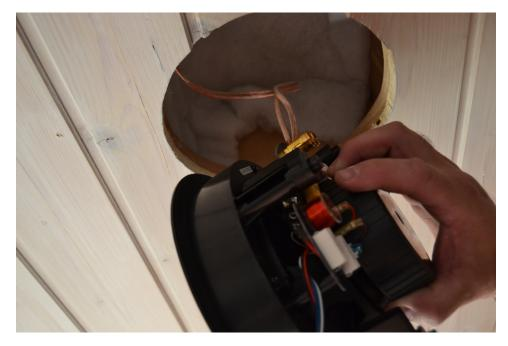
Fig 14. Speaker's terminals connected by cable + to + and - to -.
