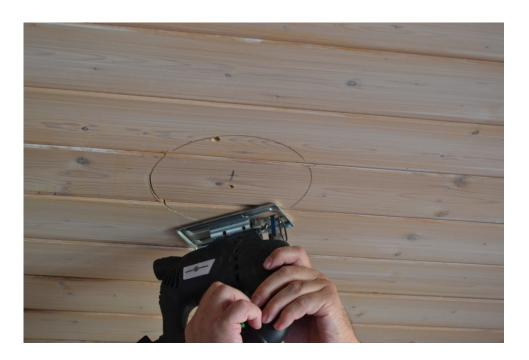
Fig 3. Cut the hole with a jigsaw.
