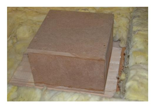
**Fig 9.** The cabinet is fitted over the hole with adhesive or sealant fitting.
