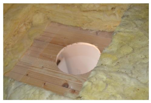
**Fig 6.** Remove the insulation in the attic where cabinet is to be placed. Remember to restore the insulation material so that it corresponds to the thickness above the cabinet as the rest of the insulation in the attic.
