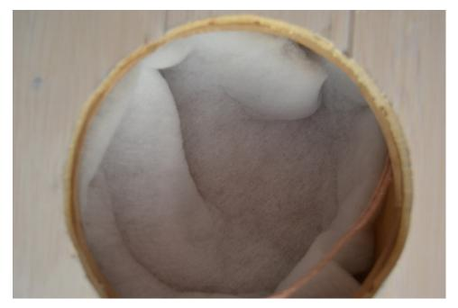
Fig 12. The insulation material is distributed loosely.
