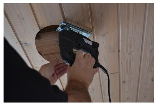
Fig 4. Carefully remove the excess material away.
