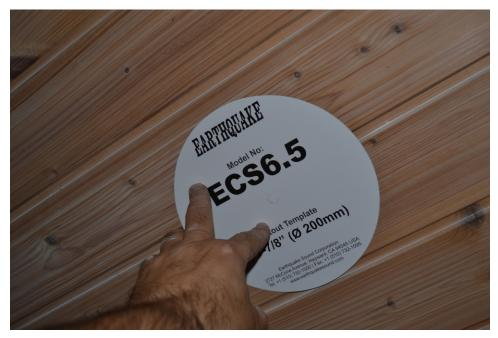
**Fig 2.** The supplied template has to be placed where the hole should be and draw a circle around the perimeter. Check on the ceiling there is no cross-send wires, rafters or studs where the hole should be.
