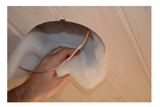
**Fig 11.** Insulation installed. Here is used Akustilux but Rockwool can also be used.
