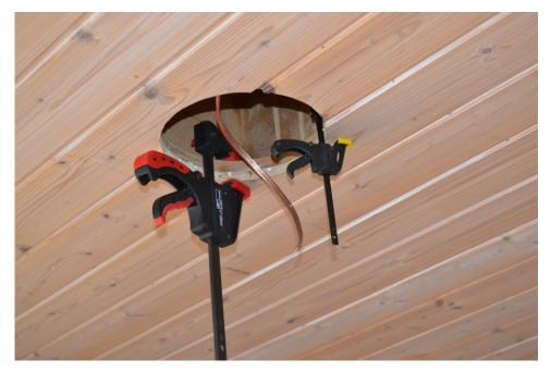
**Fig 10.** The cabinet is held by brackets until the glue or sealant has cured.
